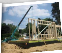
Timber Frame Work
